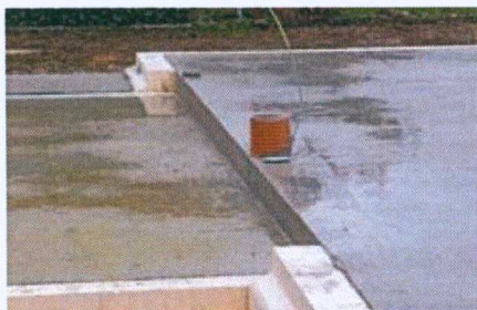
It is possible to use ISOQUICK® in buildings with different levels without creating any thermal bridges.
