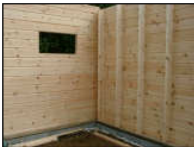
Poteaux de charpente, max. c.c. = 600
