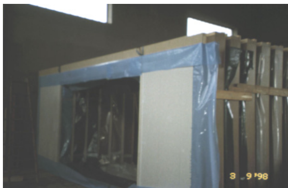
Figure 30 (left): Facade element window opening. The airtight foil joints are carefully glued, the overhanging foil is there to allow for an airtight seal with the next elements
